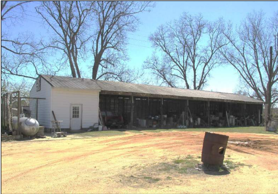
Figure 17. Maintenance shed. Northwest elevation.
