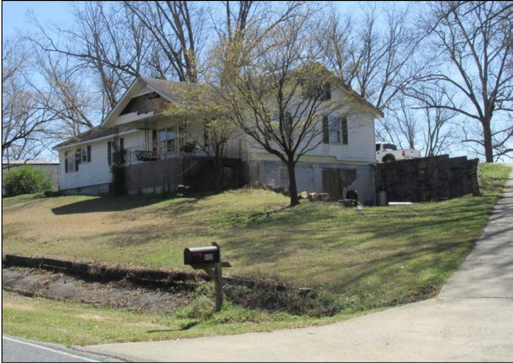
Figure 28. Front and northeast elevations of 613 Taylor Town Road.
