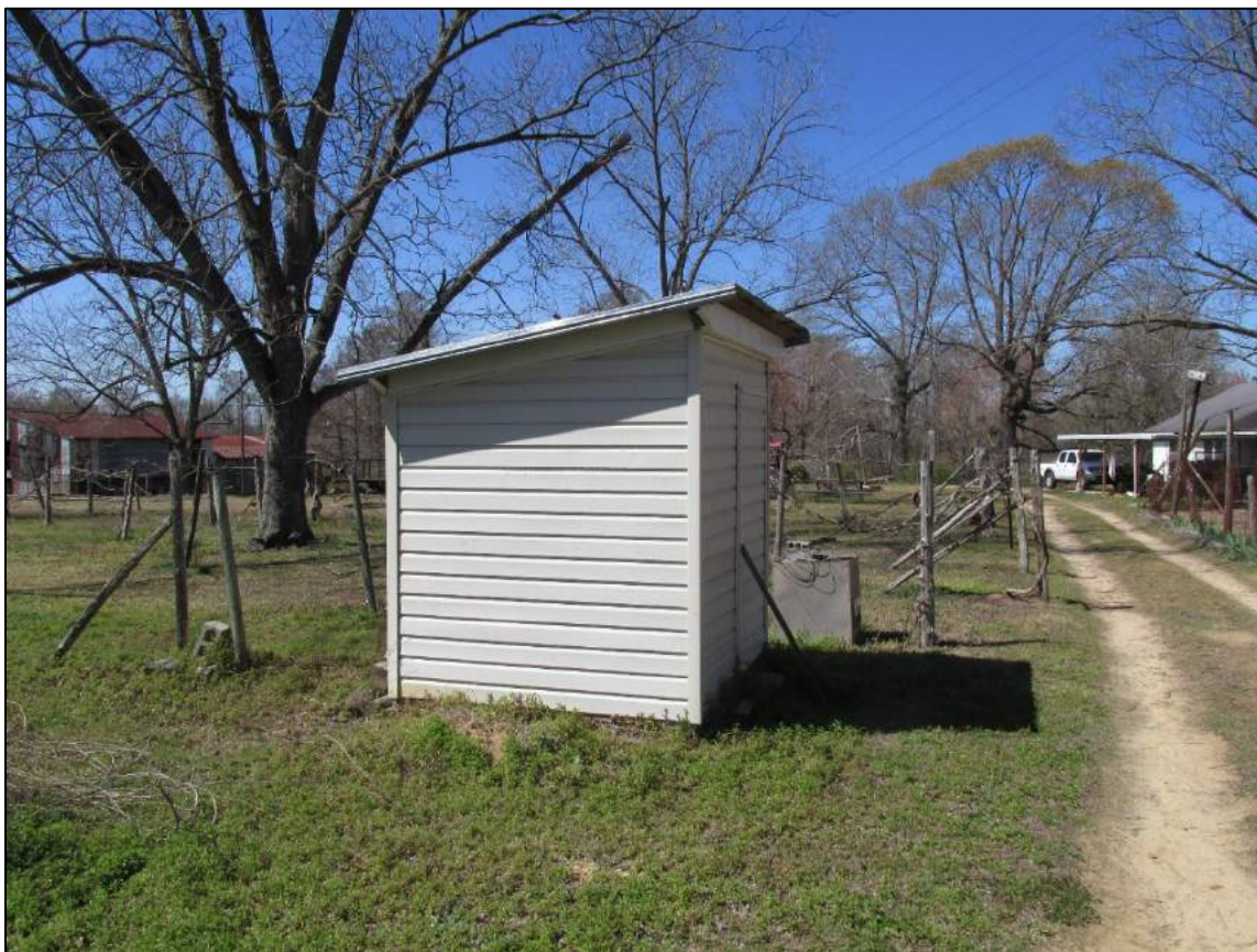
Figure 25. Pump house. Looking northwest.
