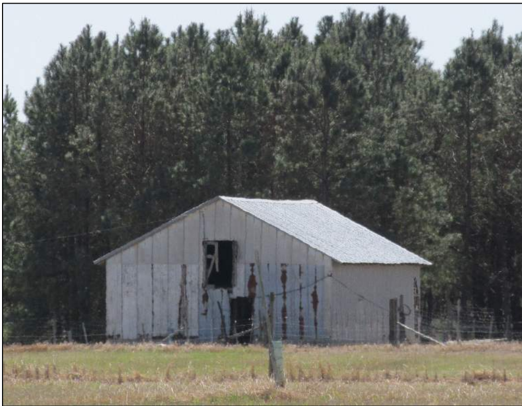
Figure 38. Barn to north of Bear Swamp. Northeast and northwest elevations.
