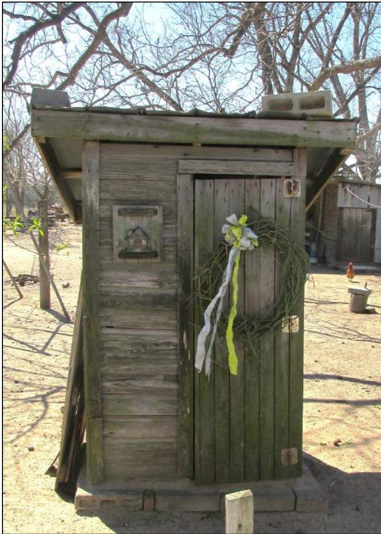
Figure 23. Former privy now used as garden tool shed. Northeast elevation.
