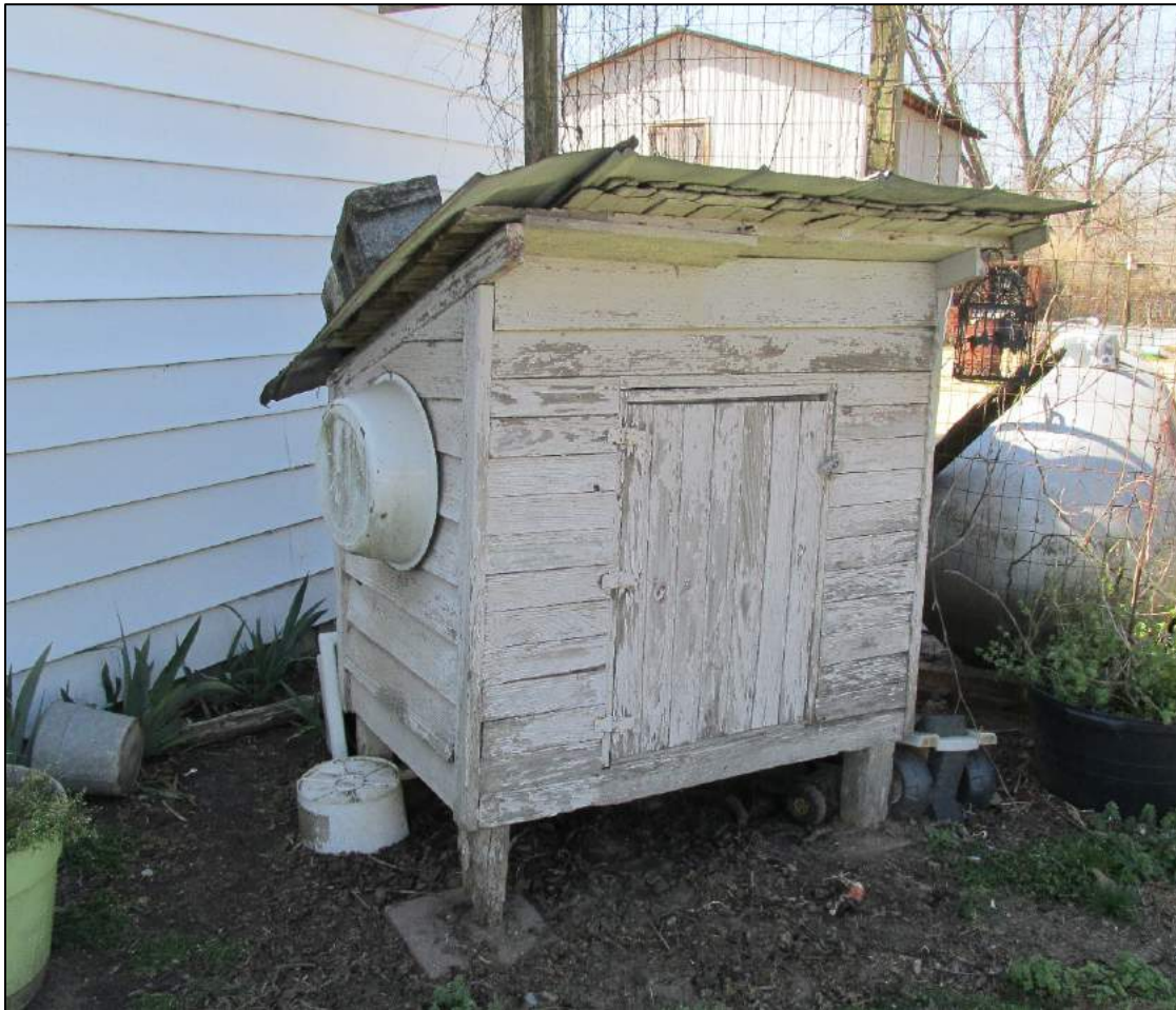
Figure 24. Milk house. Looking northwest.
