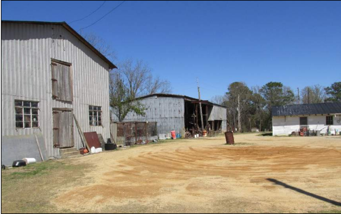
Figure 19. Yard and burn barrel between outbuildings. Looking northeast.
