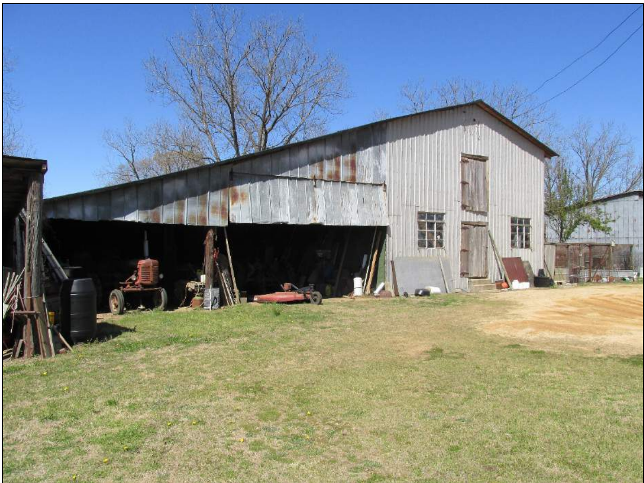
Figure 13. Pack house with shed extension. Southeast elevation.
