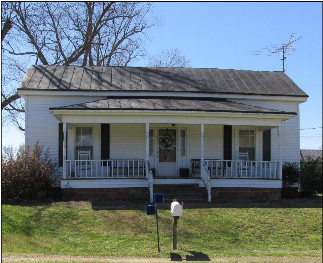
Figure 3. Ceness Taylor Farm House (597 Taylor Town Road). Main (northeast) elevation.
