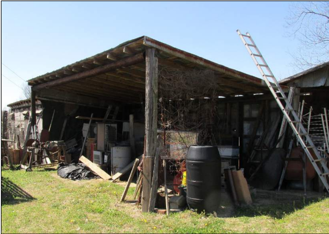
Figure 14. Pole shed. Southeast and northeast elevations.
