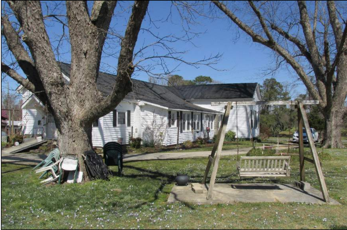
Figure 7. Rear and south elevations of house.
