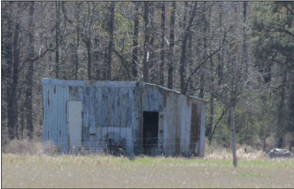
Figure 39. Former poultry house north of Bear Swamp. Northeast and northwest elevations.
