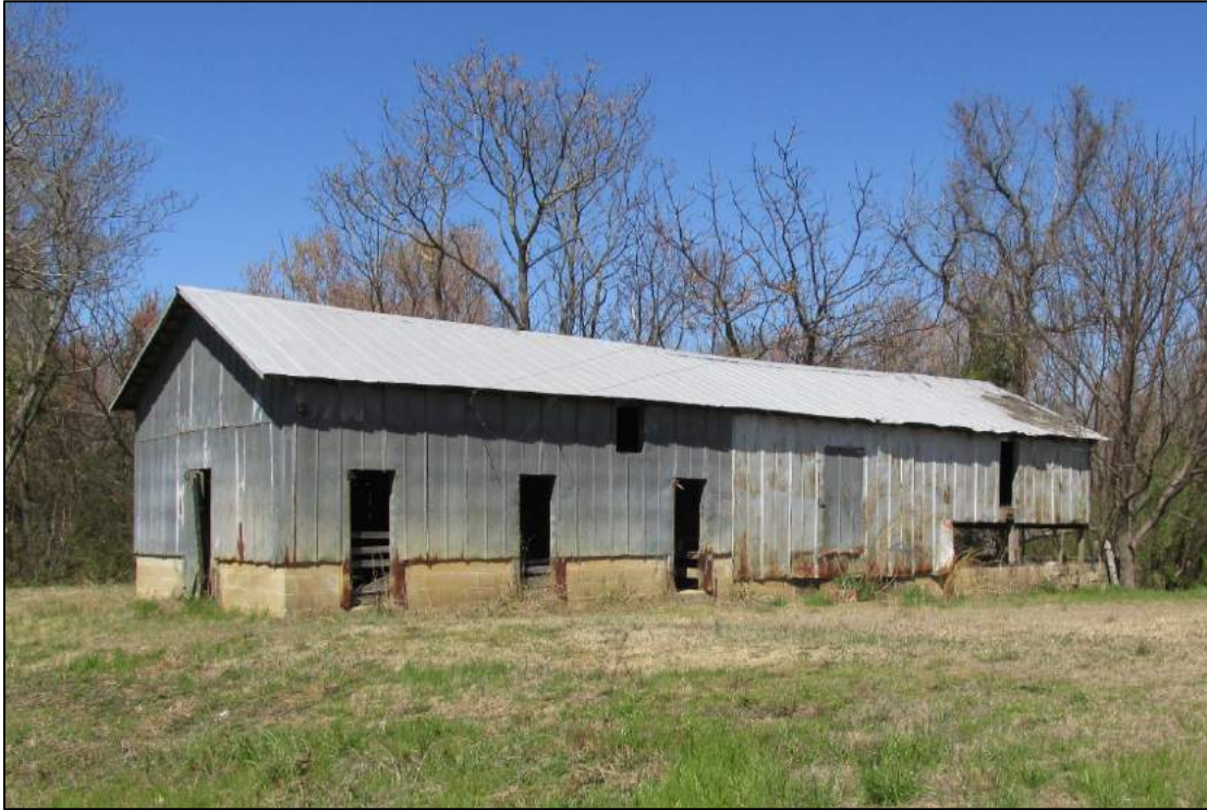
Figure 33. Hog barn. Southwest and southeast elevations.
