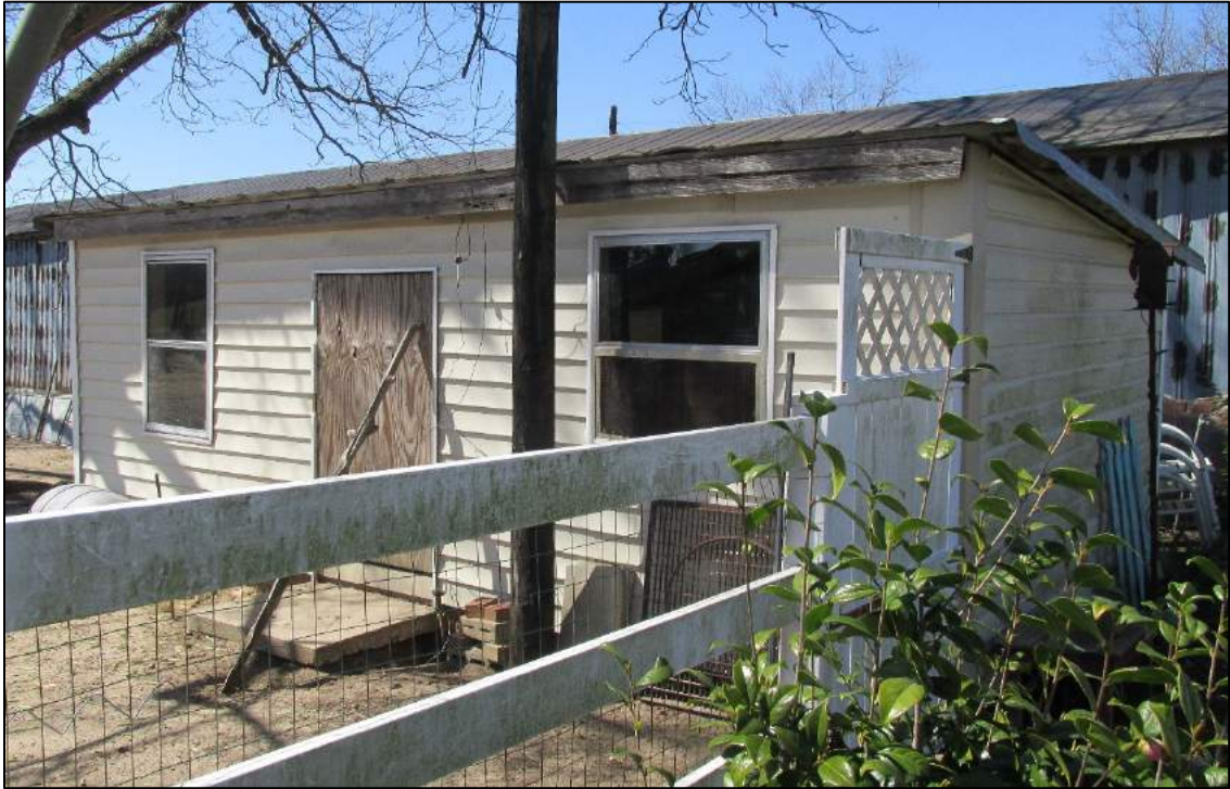
Figure 22. Former poultry house now used for storage. Southeast and northeast elevations.
