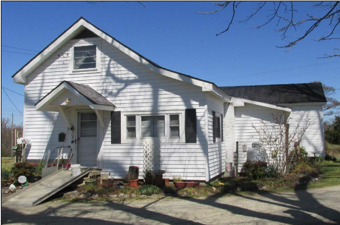
Figure 8. Rear elevation of house.
