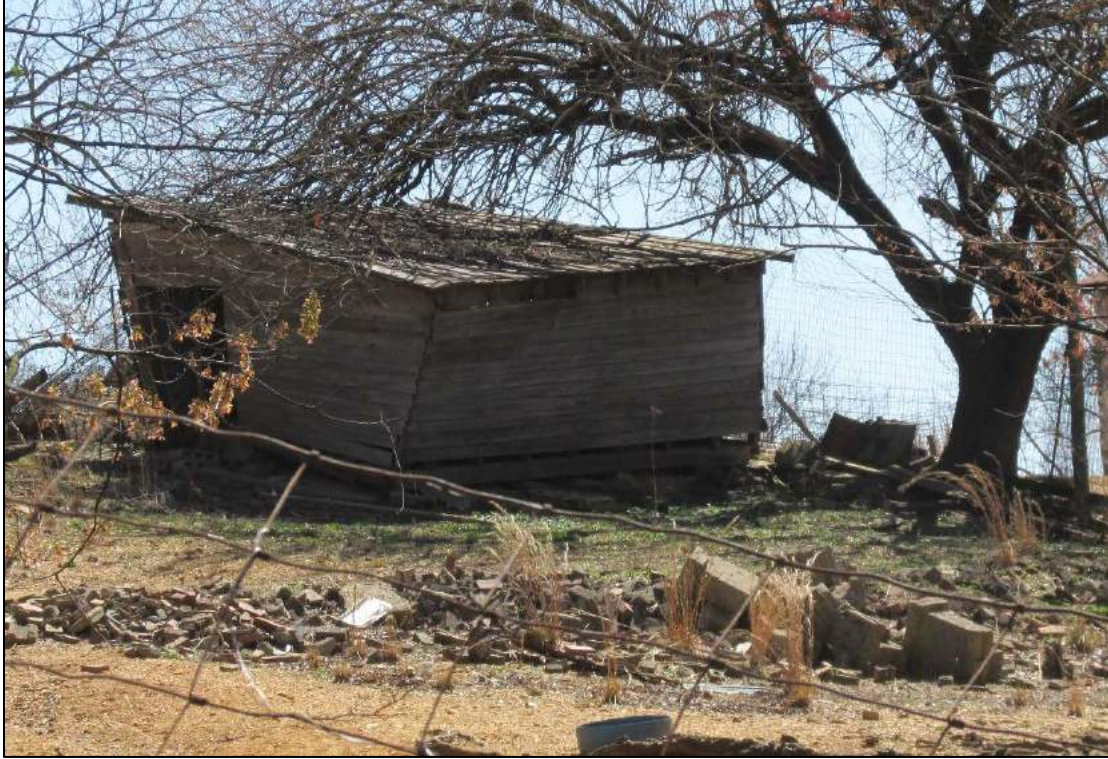
Figure 32. Poultry house by pond. North and east elevations.
