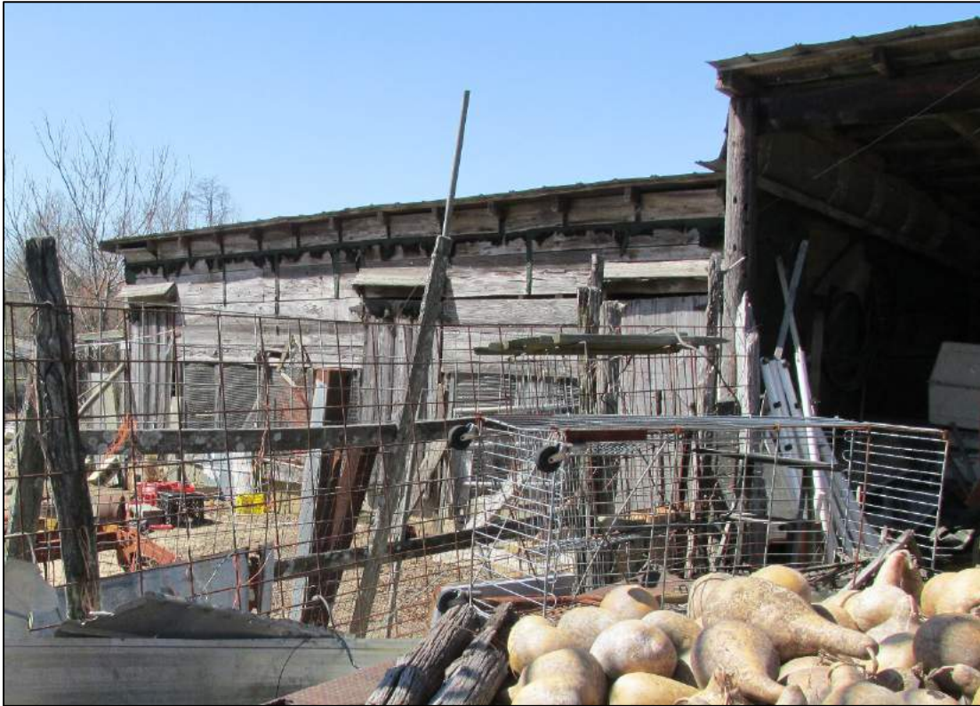
Figure 15. Poultry house. Southeast elevation.
