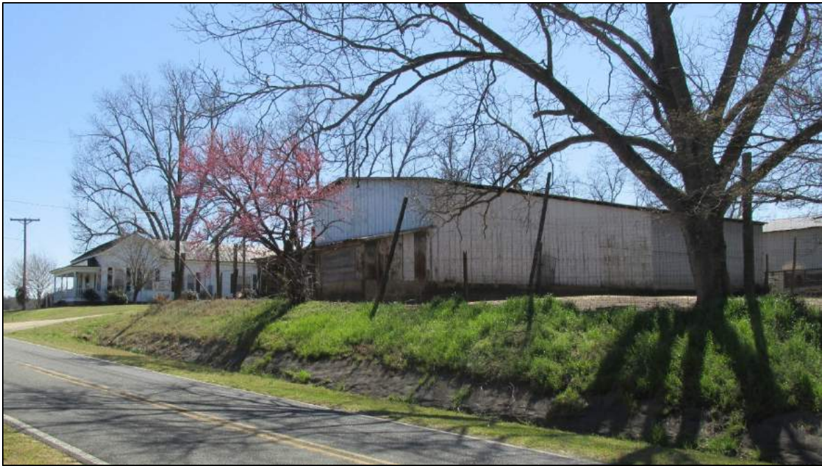
Figure 12. Barn and house on west side of Taylor Town Road.
