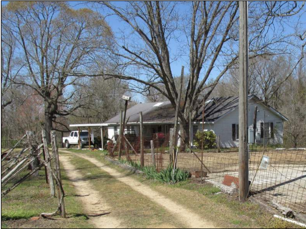
Figure 29. Rear and southeast elevations of 613 Taylor Town Road.
